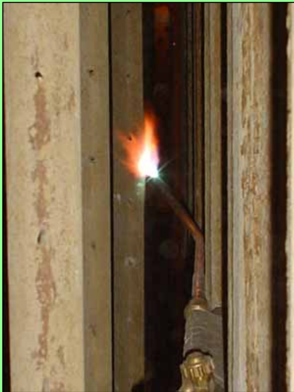
Heat Straightening RDE
